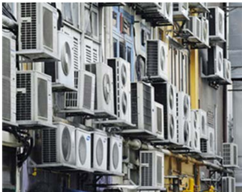
Figure 34: Anthropogenic heat from building HVAC system that is exhausted in the street canyon increases UHI effect.
